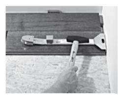
7. A pull bar or pulling iron can be used to help seat the end planks effectively
