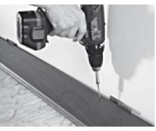
3. The planks in the first and last rows are fixed from the top with either nail or screw, the fixing is placed around 15mm from the edge of the plank
