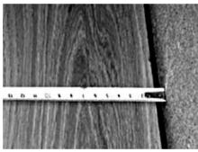
5. the last row of planks to be fitted will need to be tailor cut to suit the width left less the expansion gap. As part of preparation if the width of the room is measured and it leaves the final row to be less than 50mm reduce the front row to make it the same as the last.
