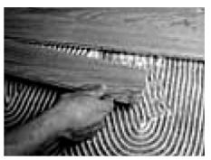
3. Set the plank into the adhesive, pressing it in making sure of a good contact and subsequent planks in a random A symmetric pattern and allowing for an expansion gap at the edge, this type of installation does not require you to glue the tongue and groove.
