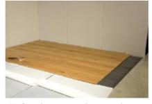
11. from here onwards, several rows can be positioned seamlessly before the protective layer between the wood and the underlay is removed
